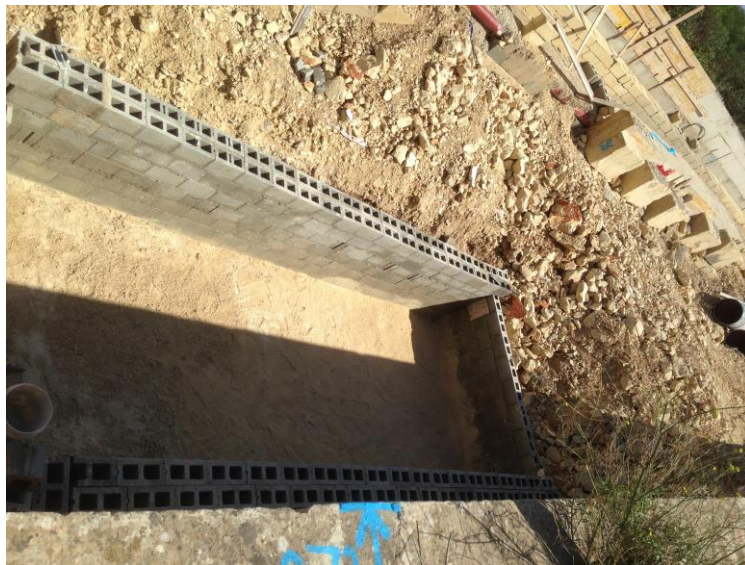
Preparation of Plinth and surrounding wall if necessary
